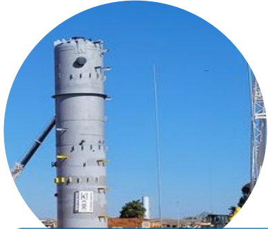
Installation of the vacuum drying tower at REPLAN
